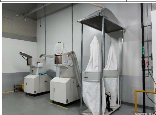
破碎废气布袋除尘及集气罩
